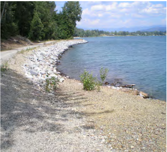
Existing riprap bank stabilization along the POBT (below).
