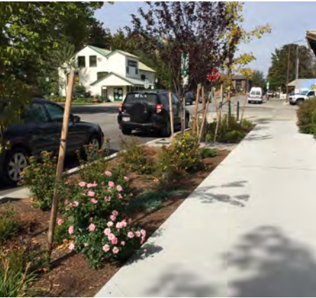
Crusher fines surface texture (top) gives the trail a natural look and feel while remaining pervious. Raingardens, such as these in Sandpoint (above), can be used at trailhead parking areas to infiltrate stormwater.
